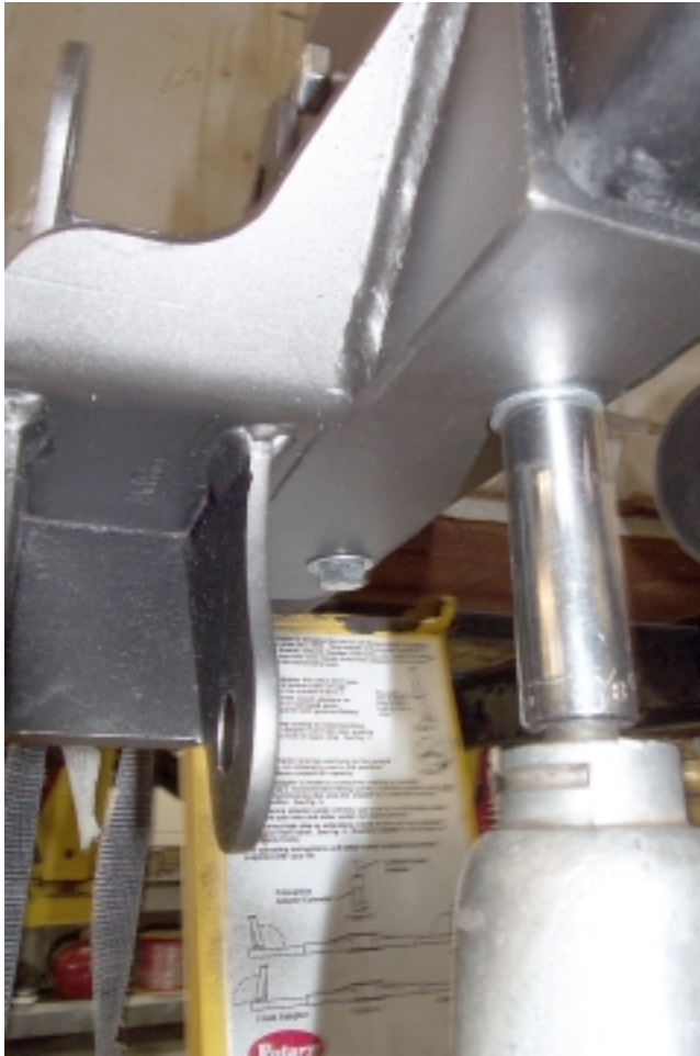
The two bolts underneath unite the bracket, frame rail and crossmember. There's no need to weld at all.
