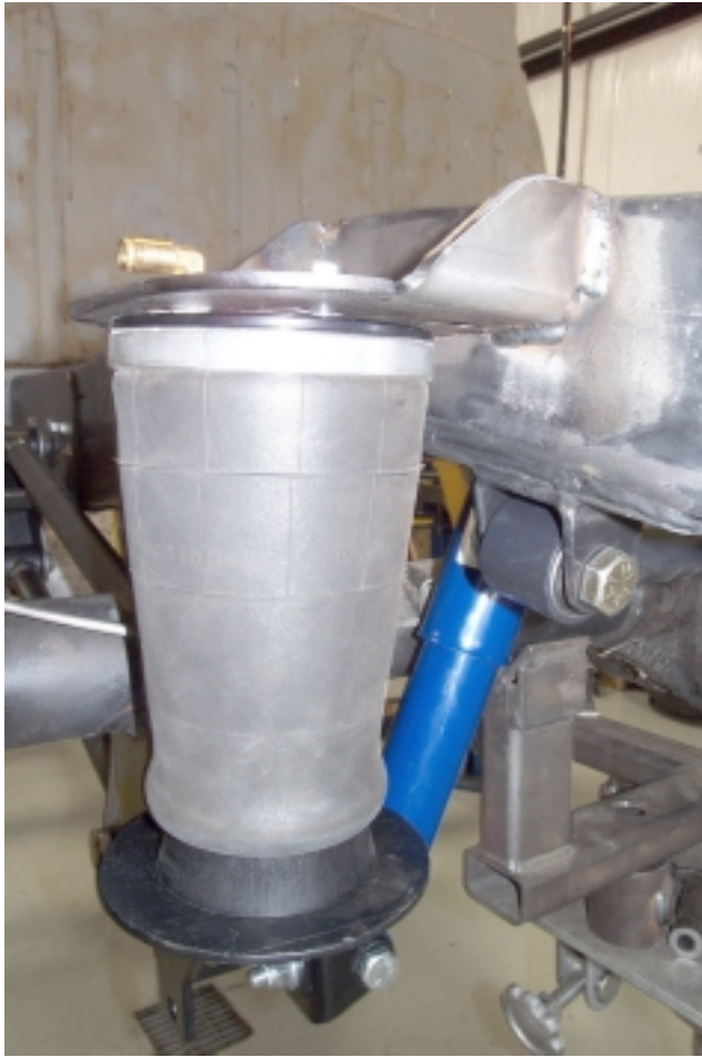
The air springs can now be bolted into place and the air lines and fittings run.
