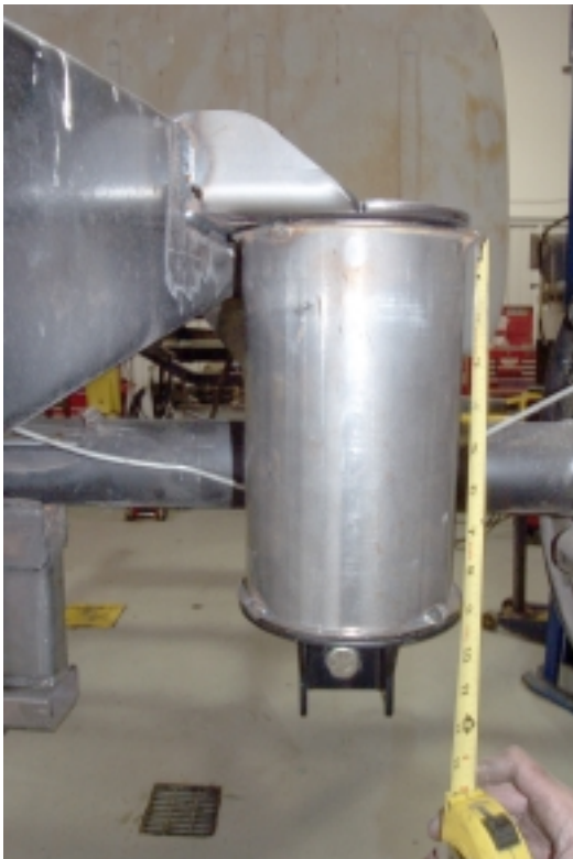
Rodney has a jig welded up for this as you can see. You can duplicate it as I did or just squarely cut a piece of 4x4 and mark centers on either end. After cutting the tack welds between axle and frame rails, reposition the axle to ride height. The top mount should be 8-1/2 inches above the lower and square with it. Because air springs have some range variation for installed height, you can add spacers to the jig if needed. Also, make sure the brackets are in alignment front to rear and side to side.
