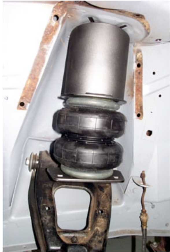
Slip the whole assembly up into the tower and into the center hole in the top mount. Leave it hang.
