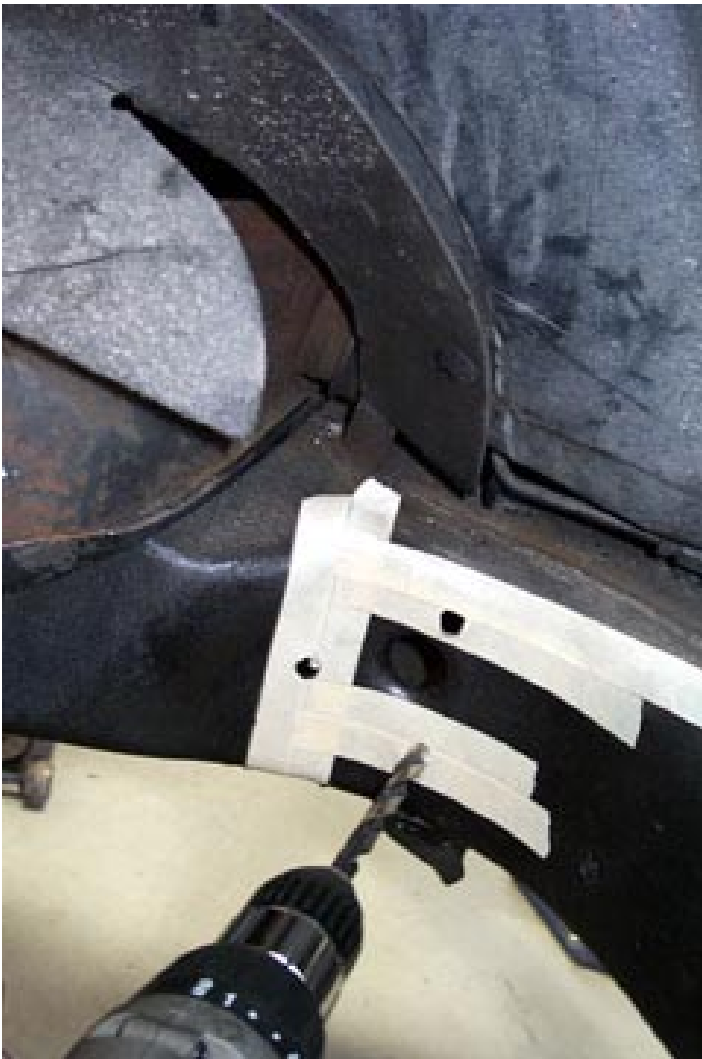
Drill the holes for the bolts with a 5/16 bit. This gives the new 3/8 self-tapping hardware the correct size hole for proper threading.
