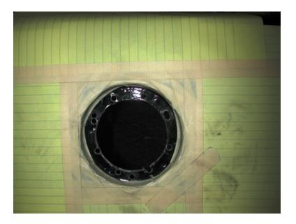
4. Remove the cap and drill the holes with a 3/16" bit.
